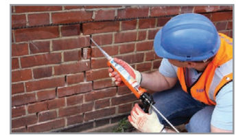
6. Re-point the mortar bed and make good the vertical crack with CrackBond TE3
