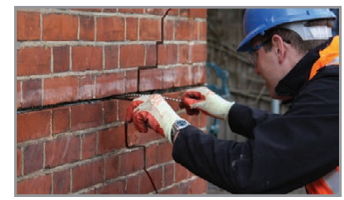
4. Using the HeliBar Insertion Tool push one HeliBar into the grout to obtain good coverage
