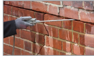
2. Clean out slots and flush with clean water and thoroughly soak the substrate within the slot
